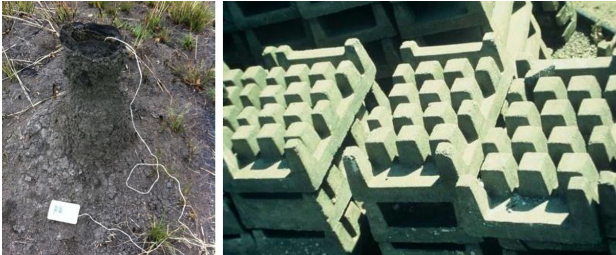
Fig. 4. Temperature measurements of termite mounds carried out by Mick Pearce (left), CC-SA-BY Licence, Mick Pearce. (b) Heat exchange floor under construction, abstraction of the biological principles of termite mounds, CC-SA-BY Mick Pearce.
